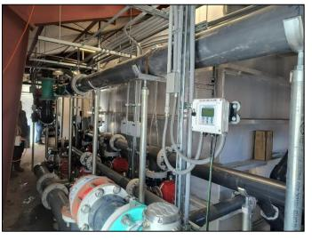
machine has been replaced with the GAC filter. A filter with GAC can remove certain chemicals and many organic contaminants from water, some of which produce odors or tastes to water. Granular activated carbon notably assists with the removal of per- and poly-fluoroalkyl substances (PFAS), which have become an increasing contaminant of concern for regulators. A GAC filtration system removes contaminants from the water supply by flowing water through the
