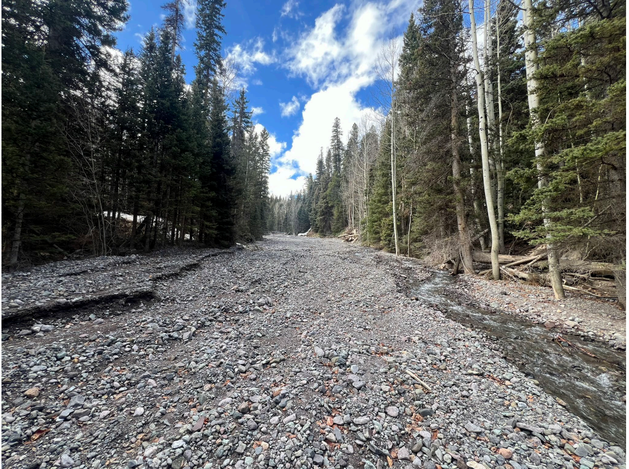
Figure 10 – Photograph showing the head cut moving up the valley approximately 700 feet downstream of the existing diversion location.
