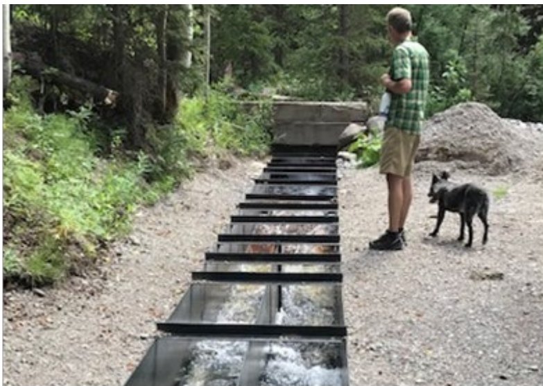
Figure 16 – Photograph of the existing sluice channel with adjustable vane.
