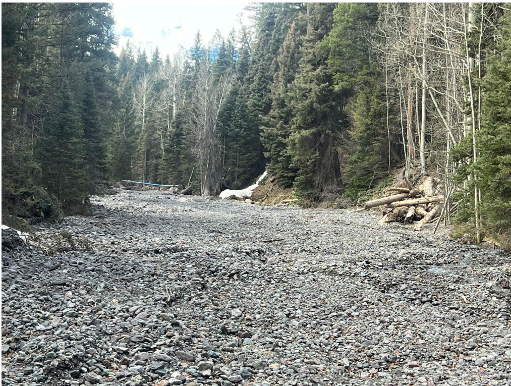
Figure 4 – Photograph showing aggradation of gravels and cobbles filling the channel.
