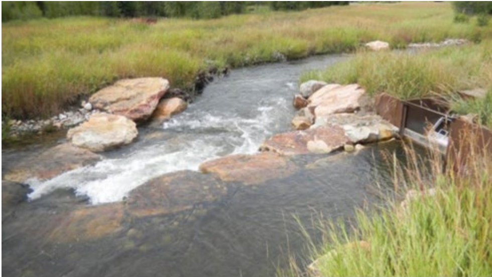
Figure 20 – Example Rock Weir with Headgate (Trout Unlimited)
