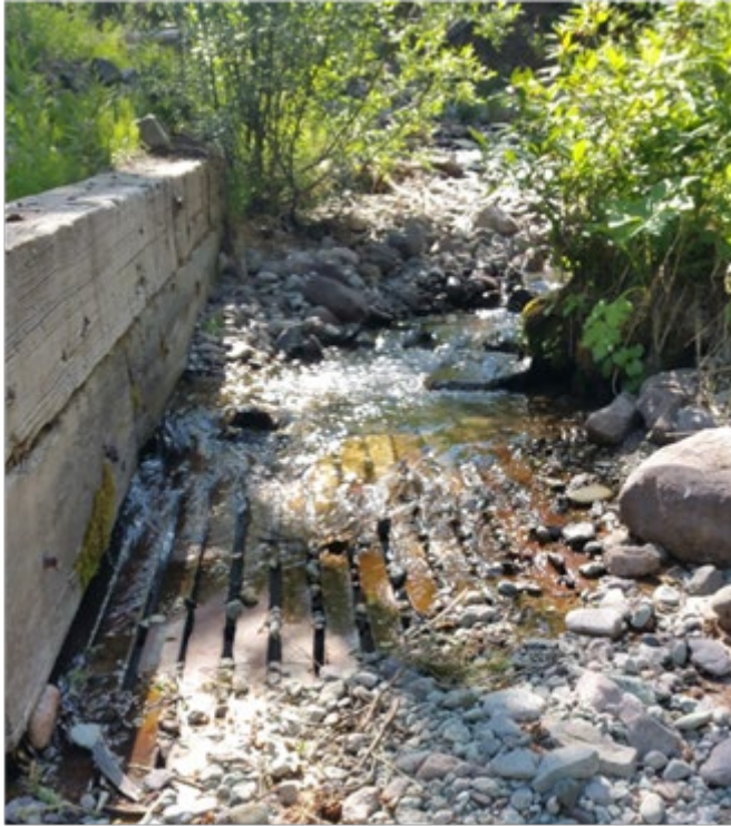
Figure 15 – Photograph of the existing intake grate structure .
