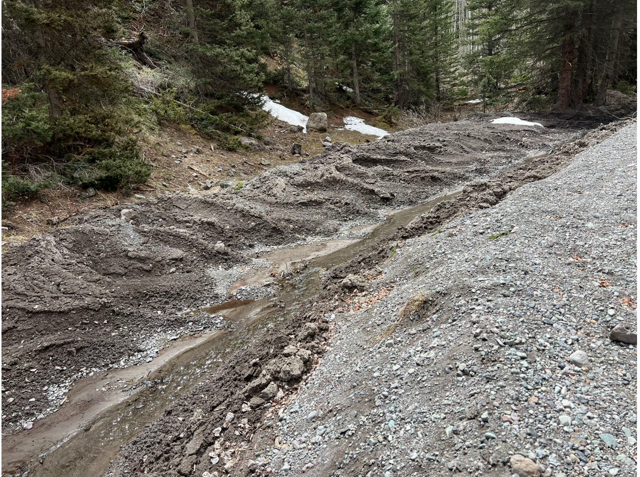
Figure 7 – Photograph showing the ditch cleaned of sand and gravel after the flood event. These materials may be reused to restore the bank as soil fill in coir wraps.
