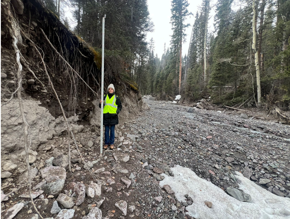
Figure 3 – Photograph looking upstream at the main channel where the channel avulsed and eroded the right bank.
