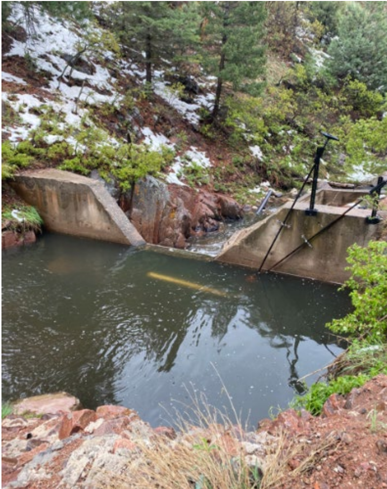
Figure 21 – Example Concrete Weir
