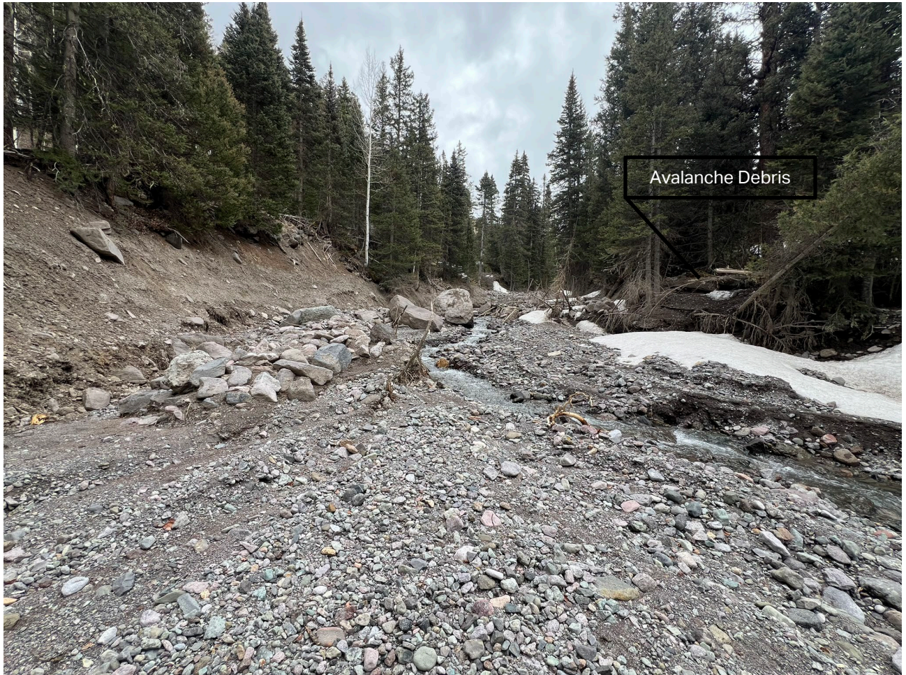
Figure 14 – Photograph looking upstream at the channel approximately 800 feet upstream of the existing diversion location.
