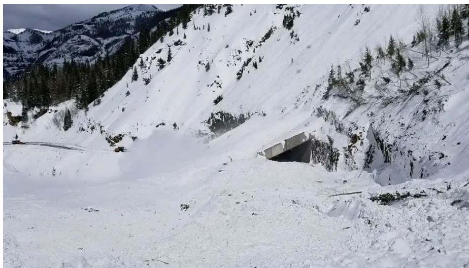
Figure 5-Avalanche at the snowshed on Highway 550
