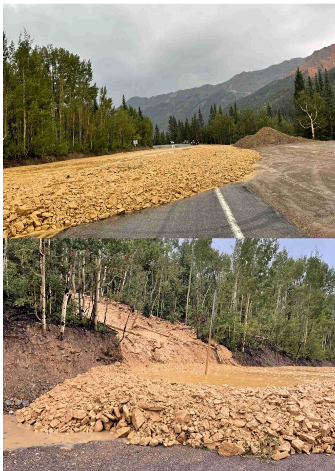
Figure 10-Landslide on Red Mountain Pass
