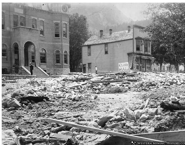
Figure 8-City of Ouray Flood 1909
