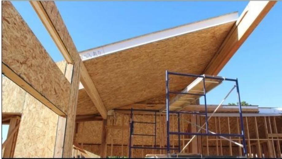
Typical beam and panel construction
