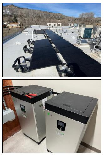
solar/storage microgrid emergency power system to provide electrical resilience to the 2,000 square foot Decker Community Room.
