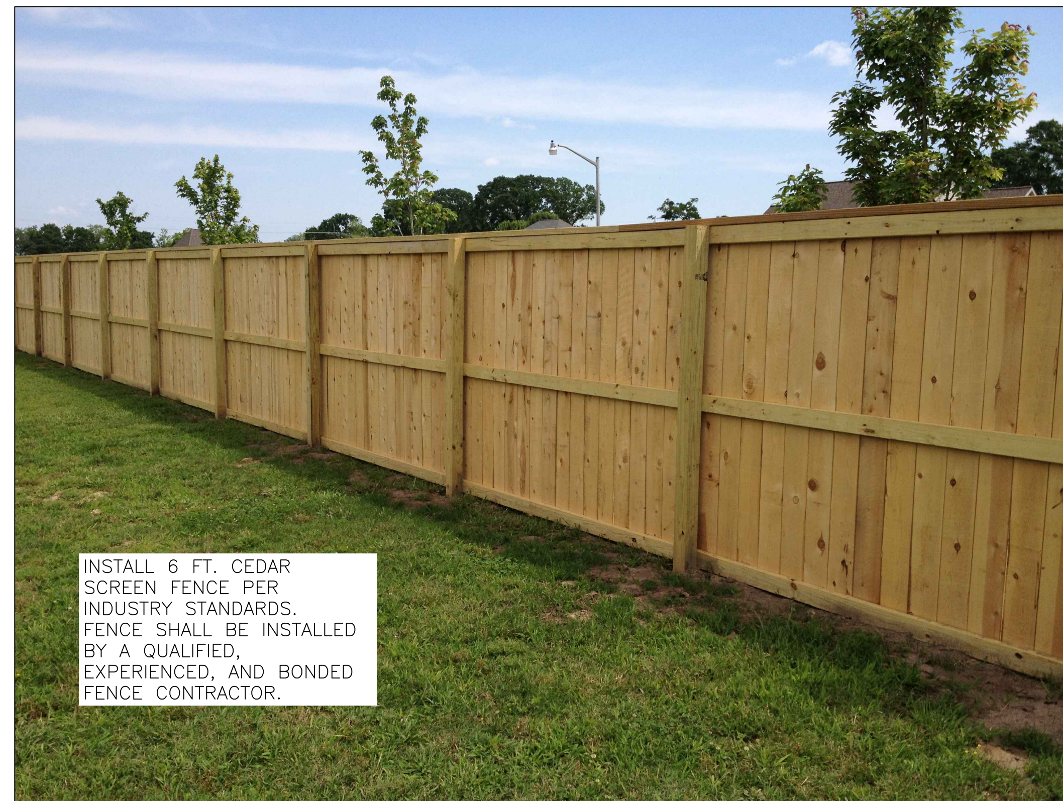
E 6 FT. TALL CEDAR SCREEN FENCE L-2 NOT TO SCALE
