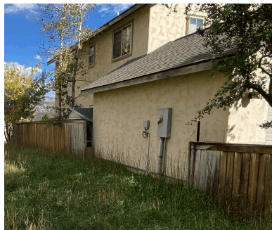
(5) 412 Amy Way fence - 4' front / 6' side yard
