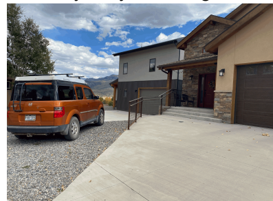
434 Amy Way fence w/handrail
