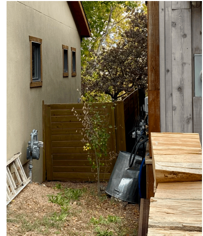
(3) 420 Amy Way - wood side yard "L" fence
