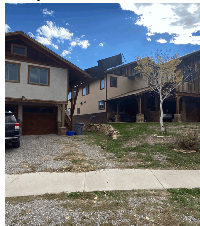
436 Amy Way retaining wall
