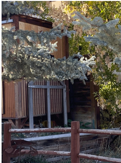
(9, con'td) 424 Amy way - second side yard fence, abutting shed, over 5' and solid wood
