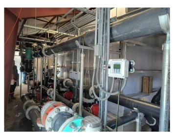
contaminants from water, some of which produce odors or tastes to water. Granular activated carbon notably assists with the removal of per- and poly-fluoroalkyl substances (PFAS), which have become an increasing contaminant of concern for regulators. A GAC filtration system removes contaminants from the water supply by flowing water through the GAC material, which pulls the contaminants like PFAS out of the water and forces them to stick to the filtration media.
