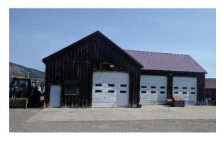
concrete slab on grade floor. Manufactured wood roof trusses make up the roof structure. Walls appear to consist of 2X6 bearing wall framing with external wall girts and rustic wood siding. While the majority of the structural elements were not visible, the structure appeared to be in good condition.
