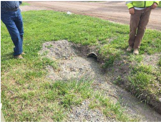
Figure 2-3. Culvert with accumulated sediment
