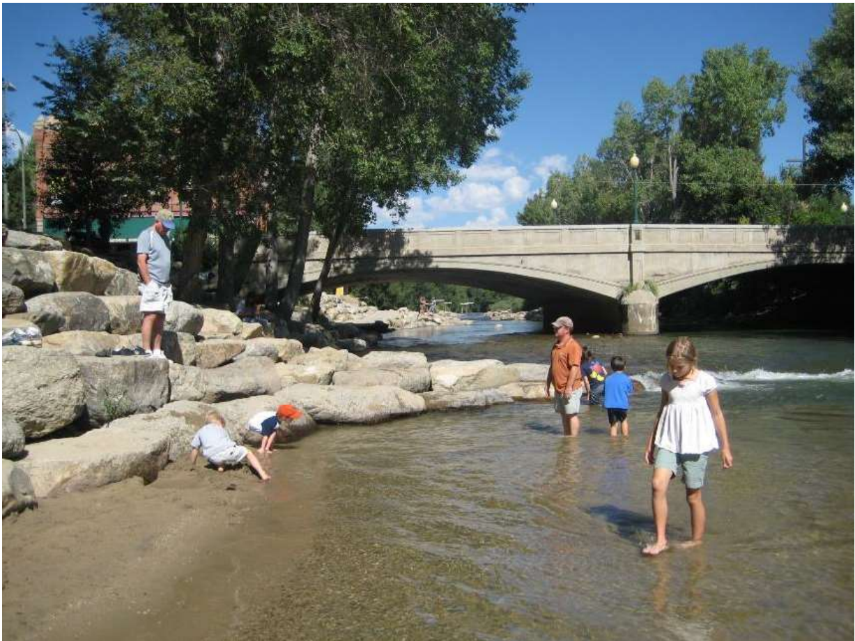
Figure 3-12. Example bank stabilization with recreation access
