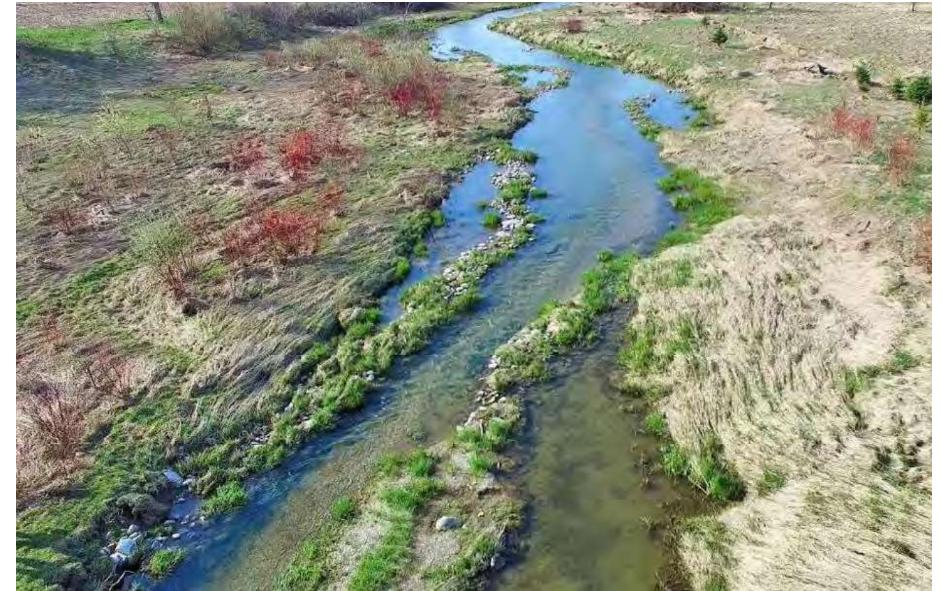
Figure 4-15. Low flow channel with native vegetation. The existing drainage in Ridgway Athletic Complex could be enhanced with native vegetation and a soft surface trail. This adds an element of interest in the park while also creating a pedestrian connection from west to east.
