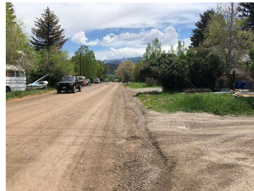
Figure 2-16. Erosion along driveways on Hyde St.
