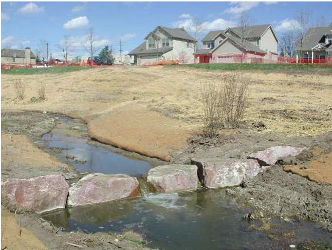
Figure 3-17. Example check structure
