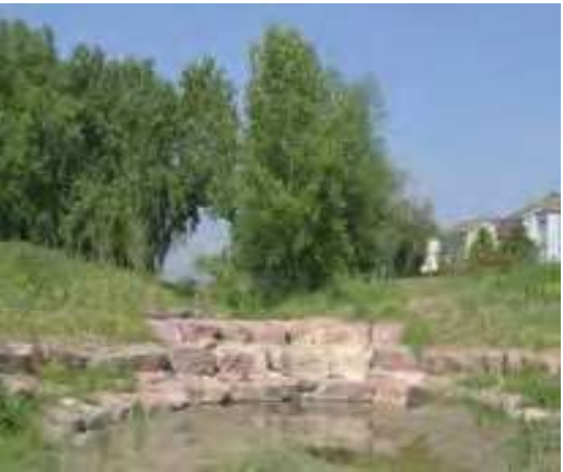
Figure 4-8. Boulder drop structure at Lilley Gulch, Jefferson County, provides channel stabilization, energy dissipation, habitat improvement and an easy way for park users to access the creek.
