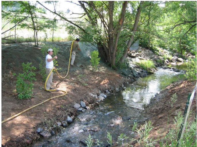
Figure 3-18. Example of bank stabilization and seeding
