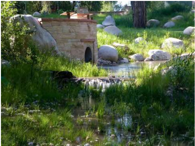
Figure 4-3. Example of a headwall incorporating an over- look with educational signage. Created wetlands are below the outfall.
