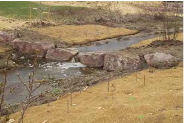
Figure 4-7. Smaller scale boulder drop structure incorporated with bank stabilization.
