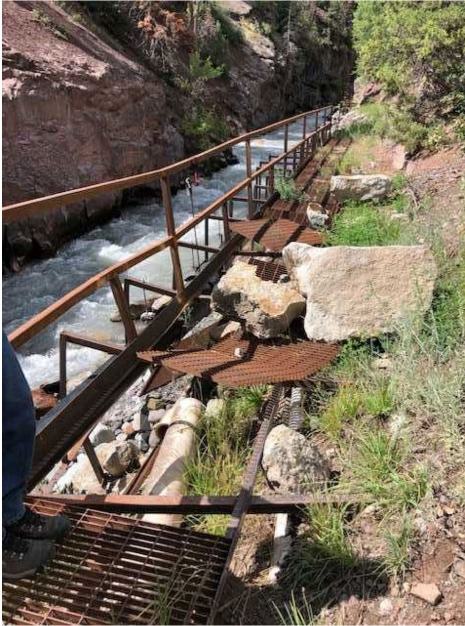
Figure 4-43 Rockfall Impacting the Ouray Hot Springs
