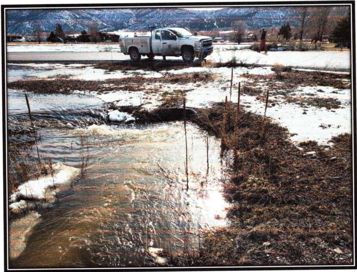
March 2019 - Very high flood water... Major snow melt off & rain combination... water was getting backed-up because this culvert under road was being blocked by slow moving water – not draining because the channel grade to the west (as seen in next picture ) is not adequate and has not been maintained in over 12 years.
