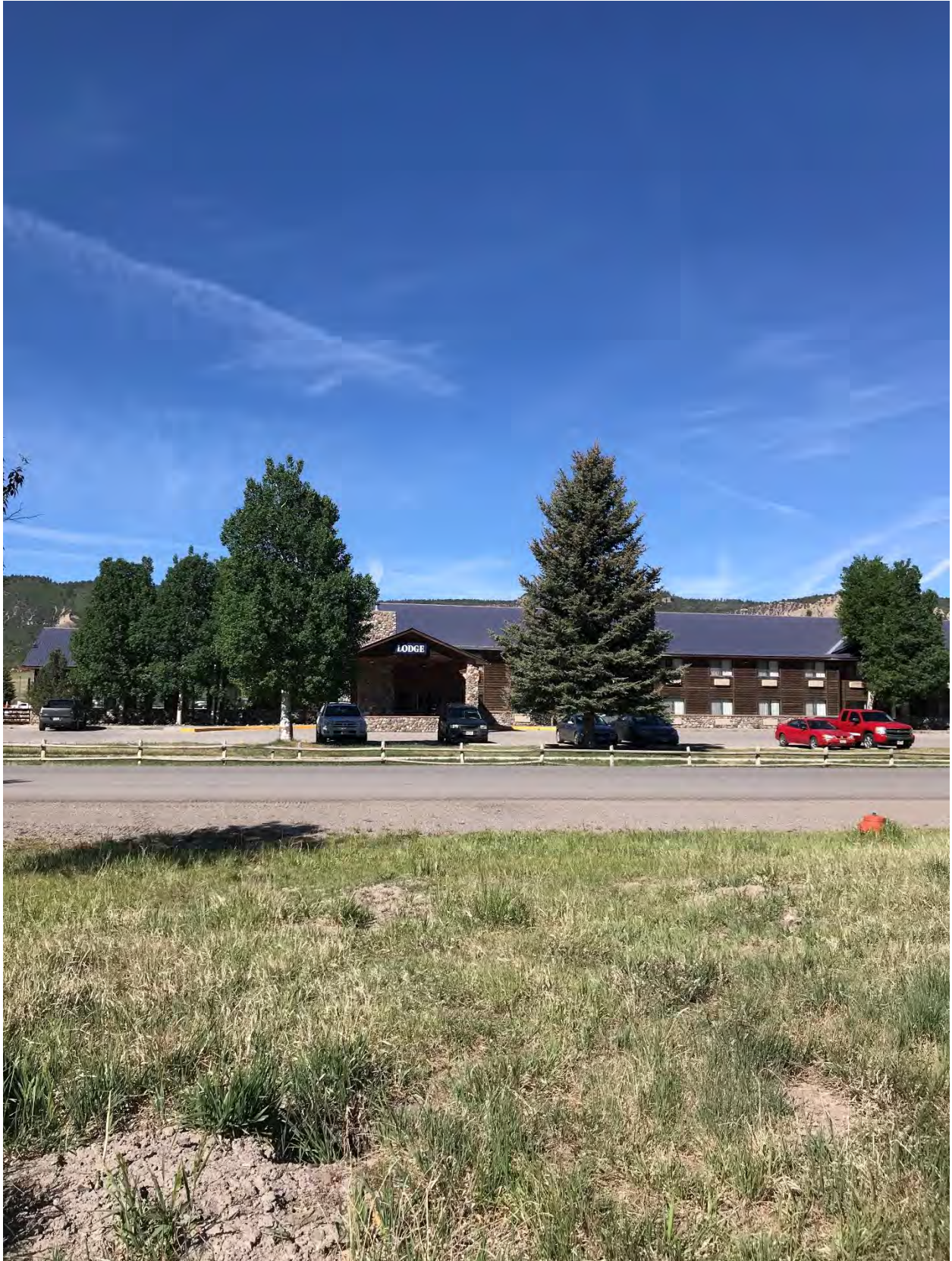
Exhibit C-1, SW corner of property looking West
