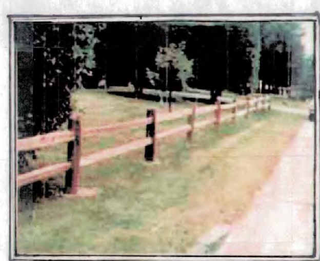
SPLIT RAIL FENCING TYPICAL W/ 2 HORIZONTAL RAILS
